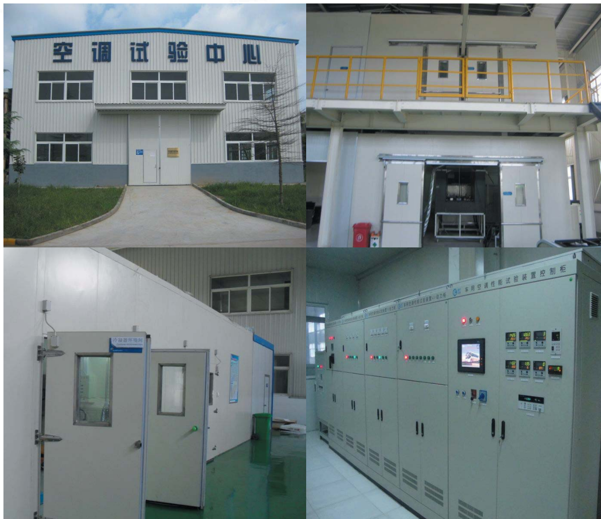
GUCHEN A/C TESTING CENTER
